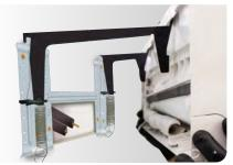
After checking WIZ brackets are firmly fastened, hook the evaporator unit to the WIZ brackets, using the unit's proper housing grooves.
